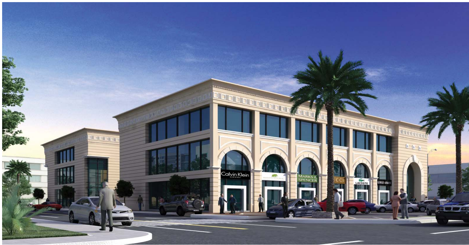
COMMERCIAL CENTER (P-076) JEDDAH, K.S.A.
