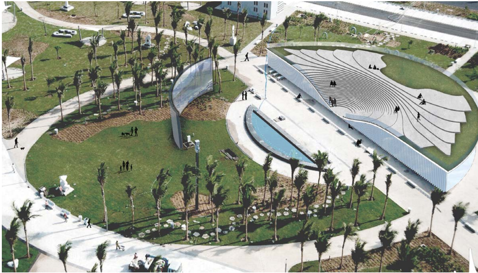
COMMERCIAL (P-617.1 C09) JEDDAH, K.S.A.
